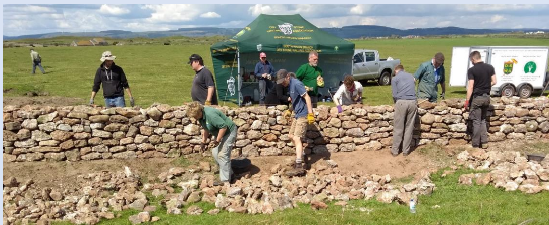
Figure 1 Dry Stone Walling © BCBC
